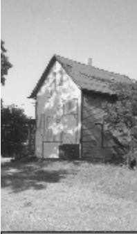
An anonymous artist's creation at the historic house on Canal Street (other side faces Howard Street)
